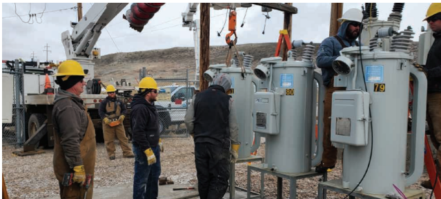
M-G crews installing new voltage regulators.
