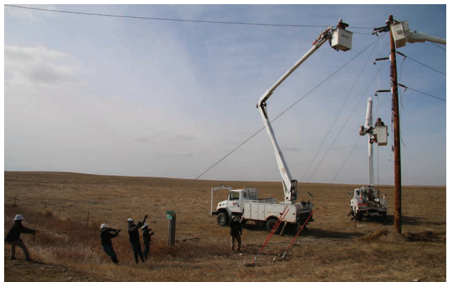
Keller Construction crews making the final connection at the Lantry transmission line move.
